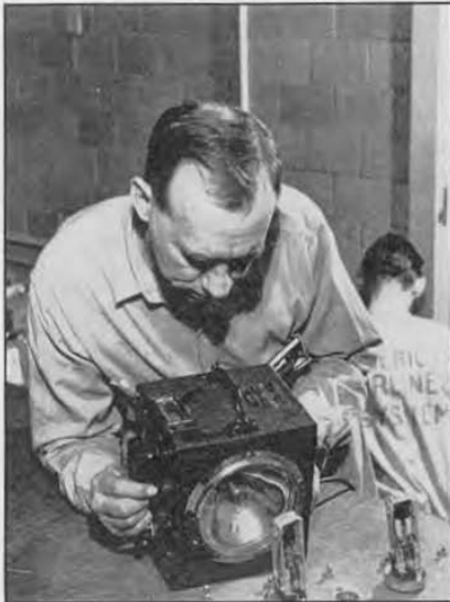
FIGURE 2. The TYPE 631-B Strobotac is used to check vibrator reeds by James Hargreaves, lead mechanic in radio-overhaul shop.
